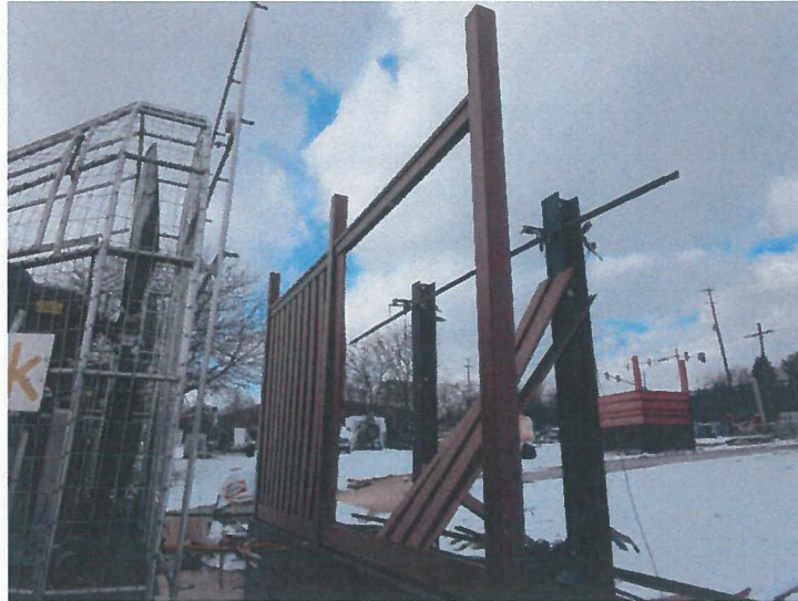
Photo No. 2 Typical Failure of Fence Assemblies
